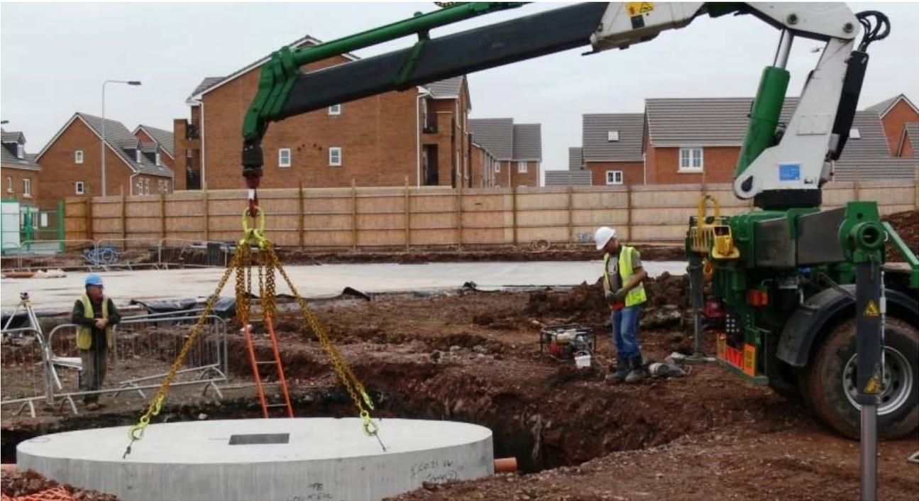
Each 23,000L precast concrete rainwater tank was placed into the final position by truck mounted crane. Only a crushed base is required and no concrete backfill. The precast rainwater tanks saved £3,000 each by eliminating a concrete base and backfill that would have been required with alternative GRP technology. The precast rainwater tanks have a standard surface load rating suitable for a 40T truck, saving additional structural design cost.
