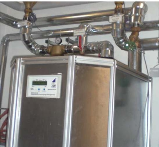
The HyproDuo is a state-of-the-art rain manager with a 300L stainless steel intermediary tank. Advanced logic control and premium Wilo pumps provide rainwater direct to WCs upon demand from the plant-room location.
