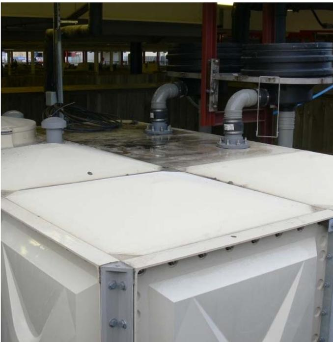
The surface mounted tank is sectional, insulated GRP with a nominal 12,000L capacity. Two stainless steel pre-tank filters remove debris from the syphonic drainage system. 800m<sup>2</sup> of the roof area was available due to the roof and drainage layout.
