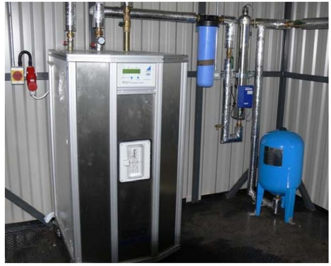
The mechanical plant room was built off-site and craned on to the roof. The rainwater is lifted from the main storage tank with a single pump to the rain manager. The rainwater is distributed from a 300L stainless steel break tank by twin booster pumps on demand to the WCs and wash down points. A fine particle filter and UV filter was specified for additional treatment.
