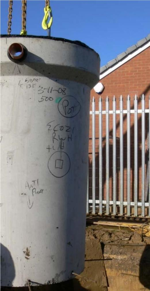
Due to poor ground conditions and uncertainty of vehicle loads on the rainwater tank surface precast concrete was specified. Precast concrete rainwater tanks are rated for 44T trucks as standard and require no additional structural works once installed. The rainwater tank was placed in the final position by delivery truck mounted crane for fast installation by Ecozi.
