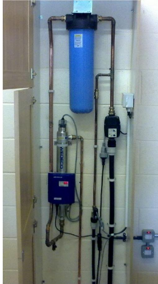
The submersible pump located in the buried rainwater tank is controlled by a flow switch located with a tank contents display panel inside the building. A fine particle and UV filter provide disinfection to the water for hand washing in the WC basin. An auto filter spray was specified to minimise routine maintenance. Every 7 days a solenoid controlled valve sprays rainwater for 3 minutes on the filter increasing the system efficiency.
