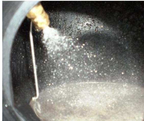
The auto filter spray operates every 7 days using rainwater to clean the filter maintaining higher system efficiencies and reducing routine maintenance. The components are pre-installed requiring simple onsite hook-up.
