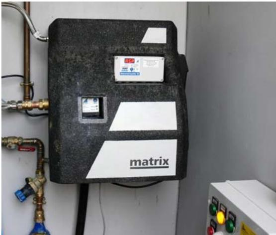
The Matrix rain manager is wall mounted in the plant room. Requiring just plumbing pipe hook-ups and two plug and socket electrical connections the Matrix is fast and simple to install. Future maintenance and fault diagnosis is straightforward.
